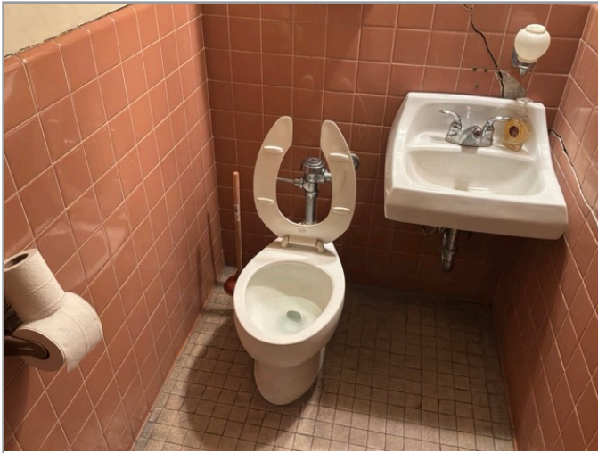
TOILET STALL OVERVIEW
