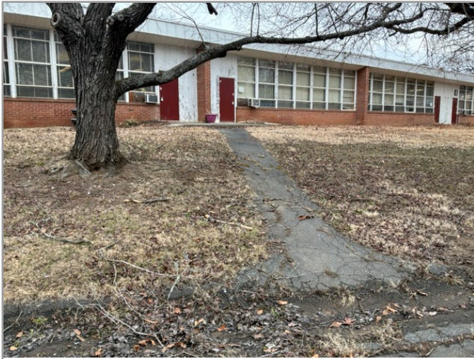
ACCESSIBLE ROUTE TO PLAYGROUND
